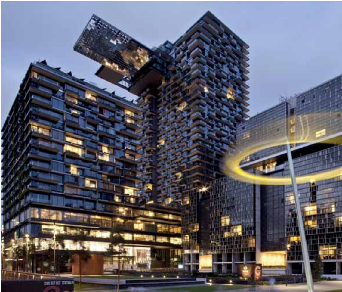
The ZCB Zero Carbon Building, designed by Ronald Lu & Partners, conceived to promote a low carbon emission lifestyle and to be a showcase of technologies to initiate a cultural change. Image is from: http://alandrealty.com
