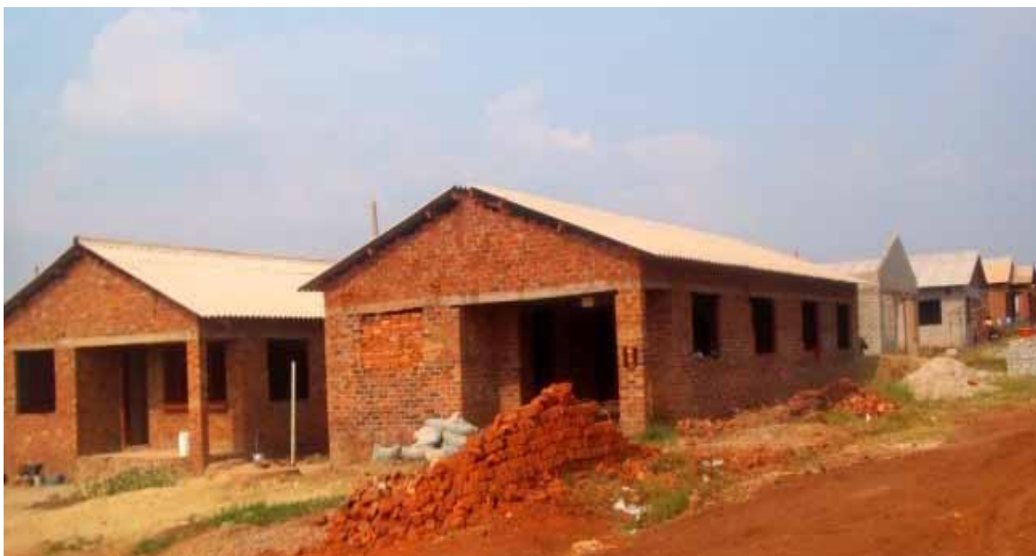
Fig. 5: Unsustainable conventional construction of houses
