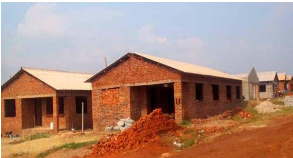
Fig. 5: Unsustainable conventional construction of houses
