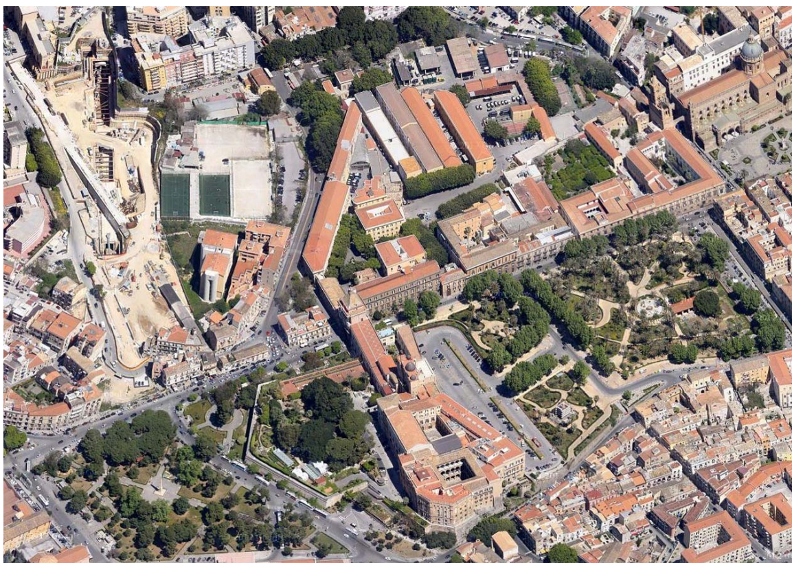
Fig. 2 The redevelopment area of Imera-Tribunale, near the Cathedral and the Regional Government Palace
