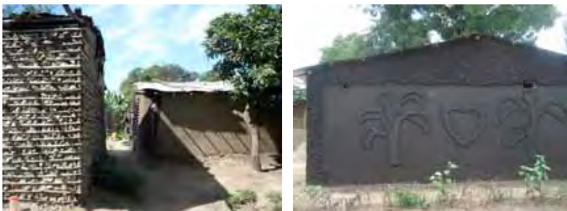
Fig. 4: Bare and plastered maticado houses (left); and decorated wall in earthen plaster 'matope' with corrugated zinc roof (right)
